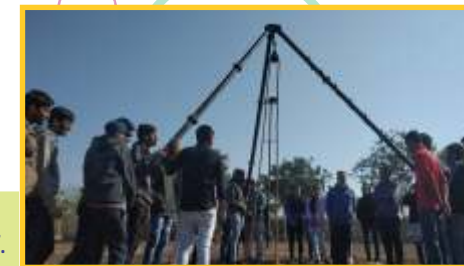
"Glance of instrument centering and leveling before commencement of test".
